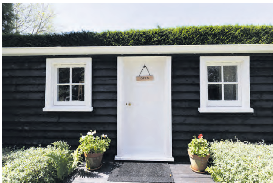
The Caboose Farm Store was created from a renovated former rabbits' hut at Beaulay Farm. PHOTOS SUPPLIED
